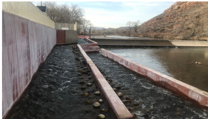
Watson Lake diversion fish passage structure: by Kyle Battige
